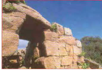
Typical entrance Entrata tipica
